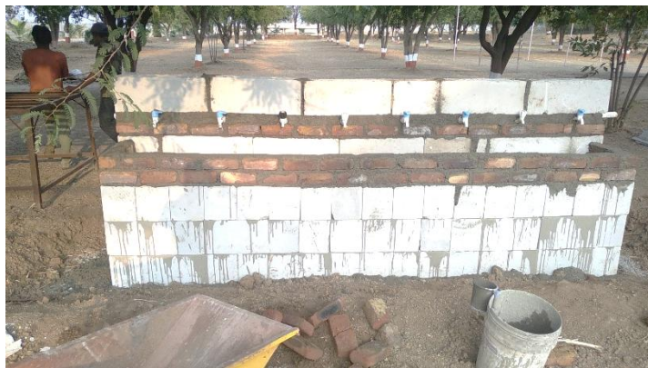
Concrete Work of Handwash Basin
