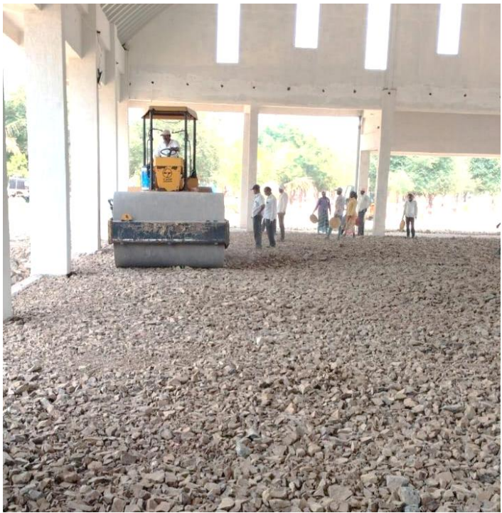
Flooring Work of Main Meditation Hall
