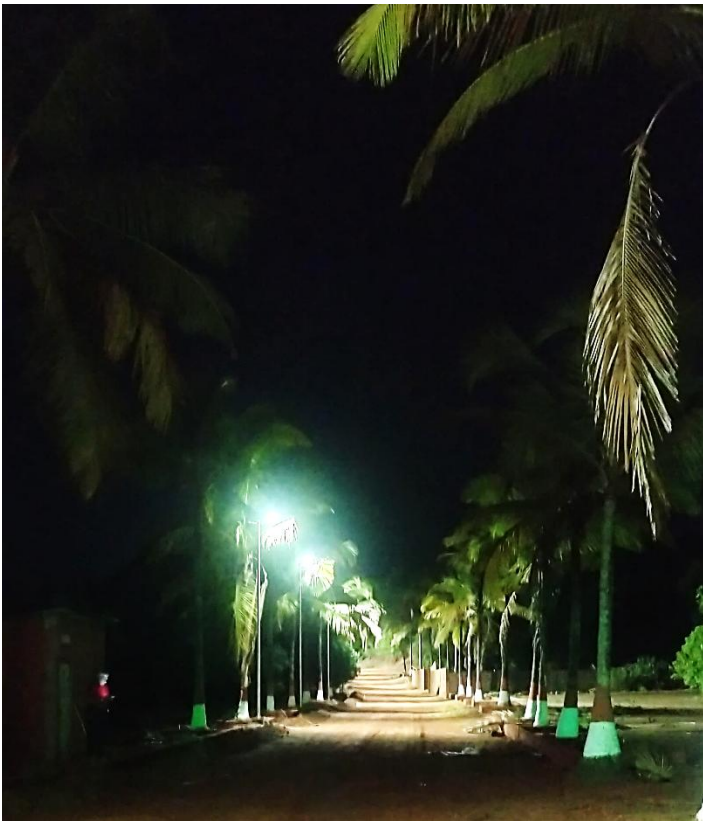
Installation High Mast and Street Lights
